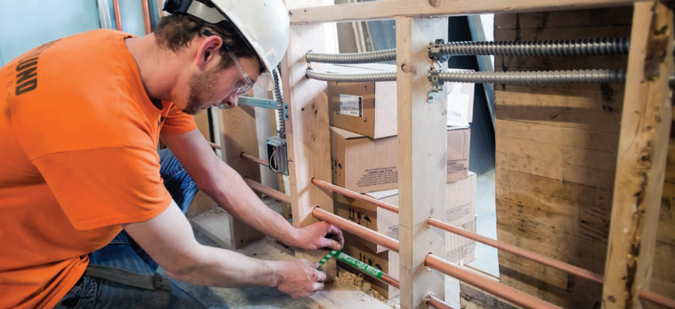
▲ Jon Bailey labels new waterlines on a commercial installation job.
