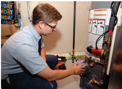
▲ Taylor Simpson works on a hot-water tank.
