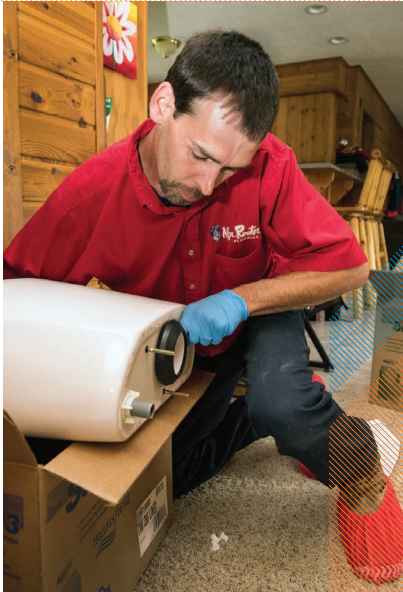
▲ Dan Biniacki installs a toilet at a residence in Hersey, Michigan.
