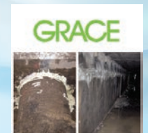
DeNeef Chemical Grouting
