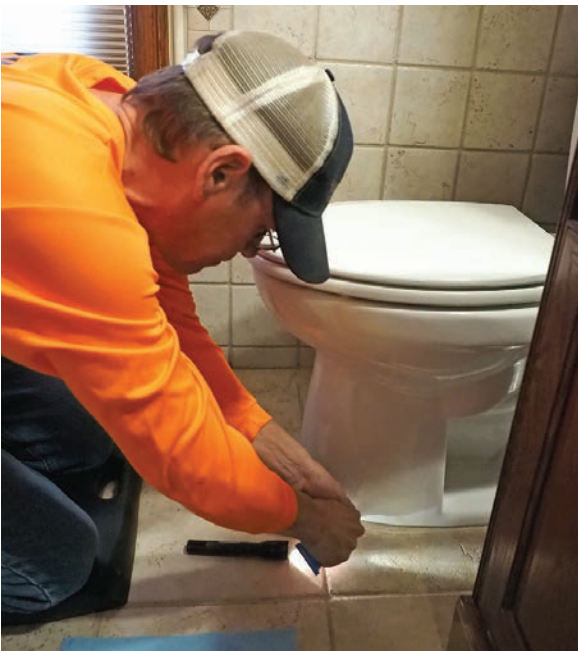
▼ Dennis Oquist reseats a new toilet.
