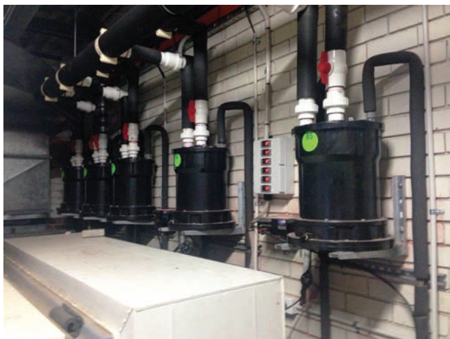
▲ Geothermal heating units sit on a wall where they are regulated to 85 degrees F. (Photos courtesy of EarthLinked)
