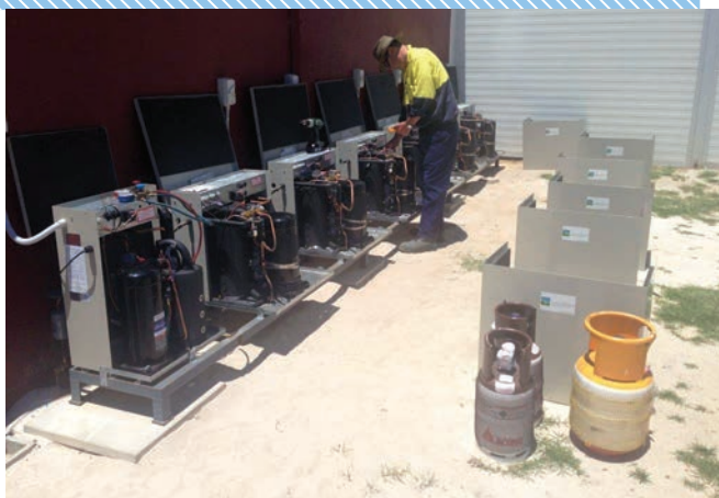
▲ A plumbing contractor checks over geothermal heating units at a pool. The units were installed on the outside wall of the pool.
