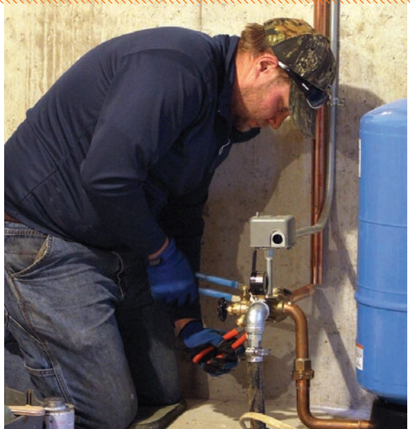
▲ Jesse Athey attaches the copper pipe to the well tank.
