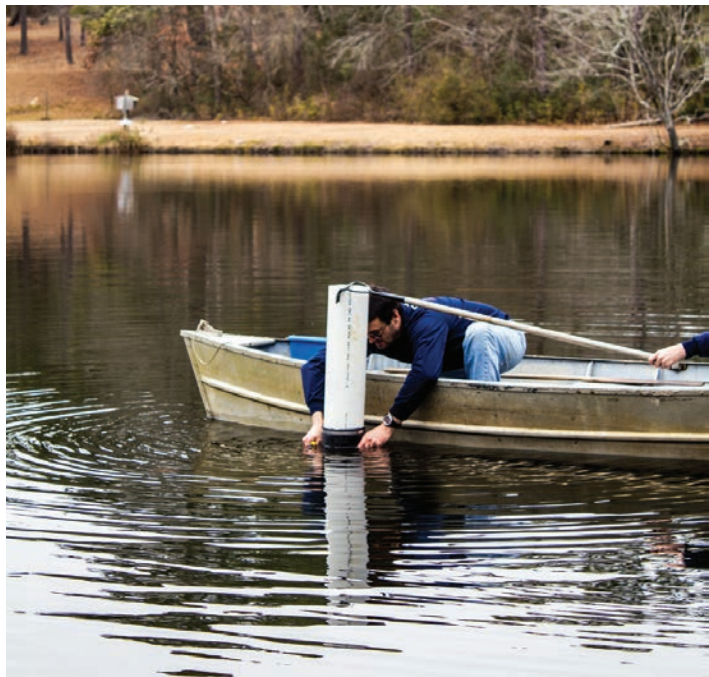
▲ Chris Bergeron of Drain Pro struggles to attach a 6-inch PVC extension with flexible Fernco coupling to a submerged cast iron overflow pipe. Jeremy Bergeron uses a bow rake to steady the extension and rowboat. (Photos courtesy of William Huang Photography)
