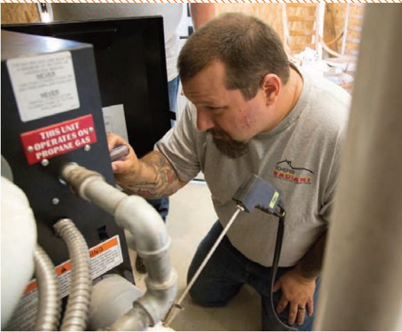
▲ Brad Schefer uses a flue gas analyzer Test Products International on a boiler system at a private residence in Middletown, California.
