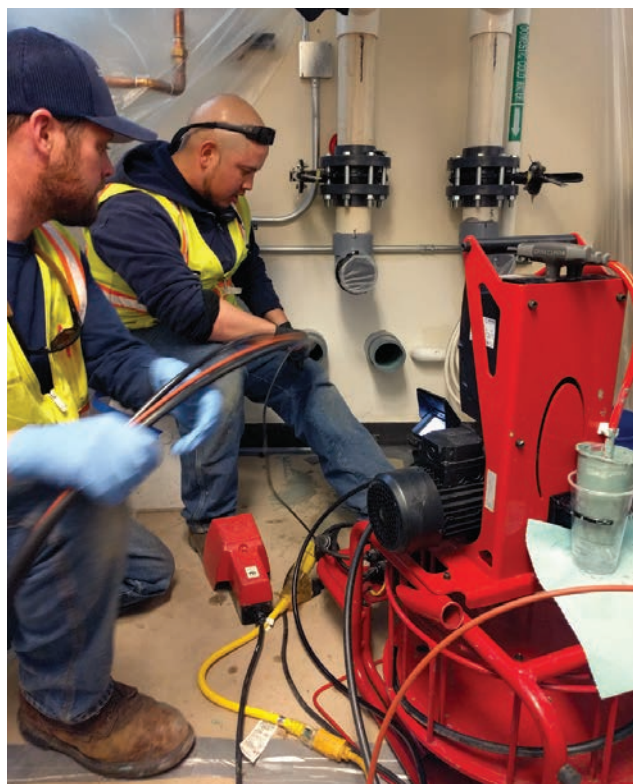
◀ Chris Tatro (left) and Ever Leon apply a coating to a cooling line at the Windsor Town Hall while watching progress on a CCTV monitor.
