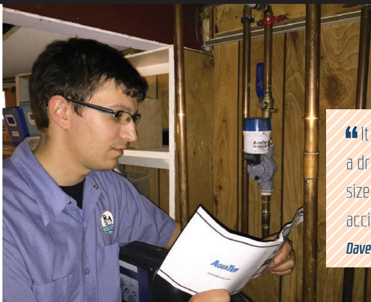
▲ DS Plumbing technician Trevor Sisson installs the AquaTrip water leak detection system from AquaTrip Pty. for a customer in Ottawa.
