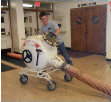
▲ Clint Spreen of SLB Pipe Solutions rolls the wetted liner into the Perma-Liner inversion tube.
