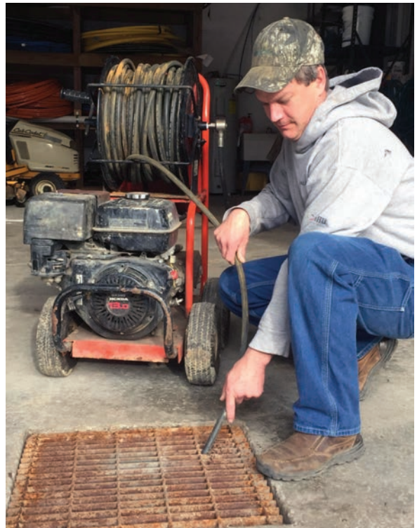
▲ David Tipton, Frazier Plumbing, Heating & Air technician, uses the company's General Pipe Cleaners J-3000 cart jetter on a job site.
