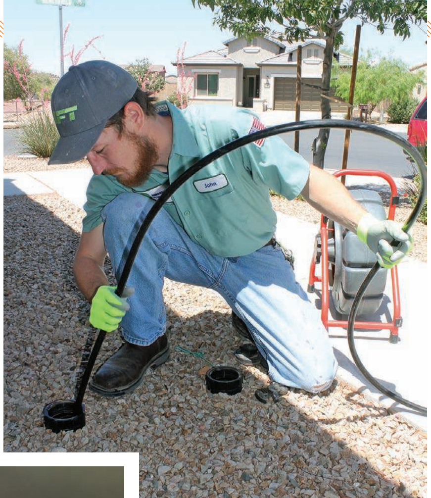
▲ John Hall, a five-year-veteran technician with Dinosaur Plumbing uses a RIDGID SeeSnake on a drain outside of a customer’s home near Tucson, Arizona.
