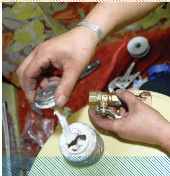
▲ Linda Hudek applies some glue to a new valve for installation.
