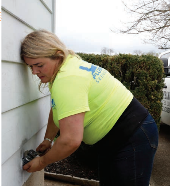
▲ Hudek tightens the packing on a hose bib at a residence.
