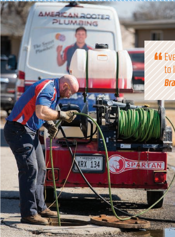
▲ Bradd Conn, master plumber and owner of American Rooter Plumbing, uses a Spartan Tool 740 Water Jet to unclog a sewer line for a client in Omaha, Nebraska. (Photography by Matt Ryerson)
