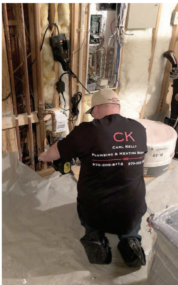
▲ Ty McLain, technician at Carl Kelly Plumbing & Heating Services, installs a FloLogic leak-sensor system at a home near Telluride, Colorado. The FloLogic device features a solid-brass ball valve that's installed where the main waterline enters a home or building. A key feature is the unit's ability to automatically shut off the water supply when it senses a leak. It's sensitive enough to detect leaks as small as 1 tablespoon of water per minute. (Photo courtesy of Carl Kelly)
