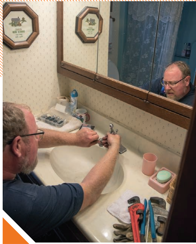
▲ Feikema disassembles a faucet for job at a residence in Munster.
