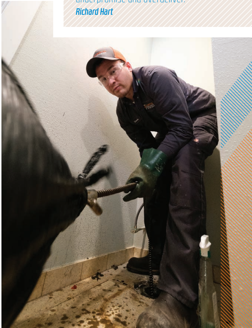
▶ Steven Shoopman snakes a sewer line in a residential remodel.
