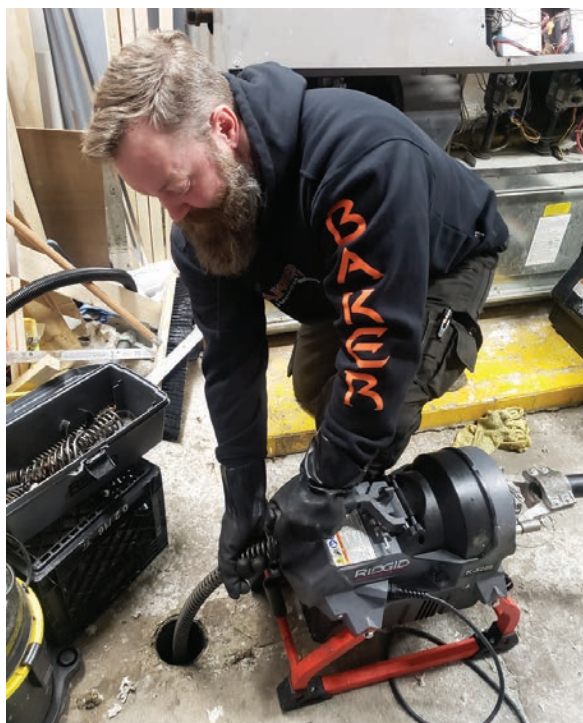
▲ Bob Baker, the owner of Baker Plumbing, Heating and Gasfitting in Calgary, Alberta, uses a RIDGID K-5208 sectional cable drain machine to unclog an 8-inch-diameter drainline in a Calgary-area hotel. (Photo courtesy of Baker Plumbing, Heating and Gasfitting)
