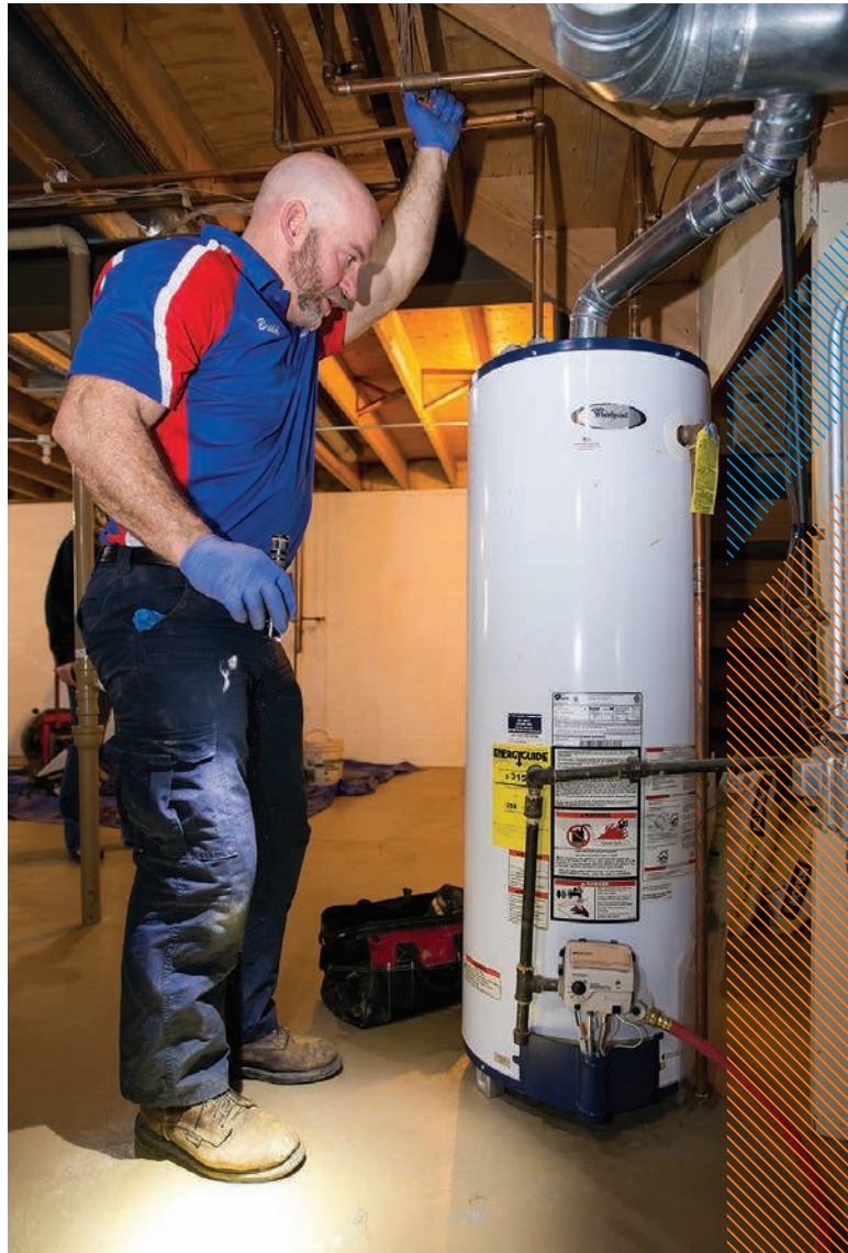
► Bradd Conn performs routine water heater (Whirlpool) maintenance.
