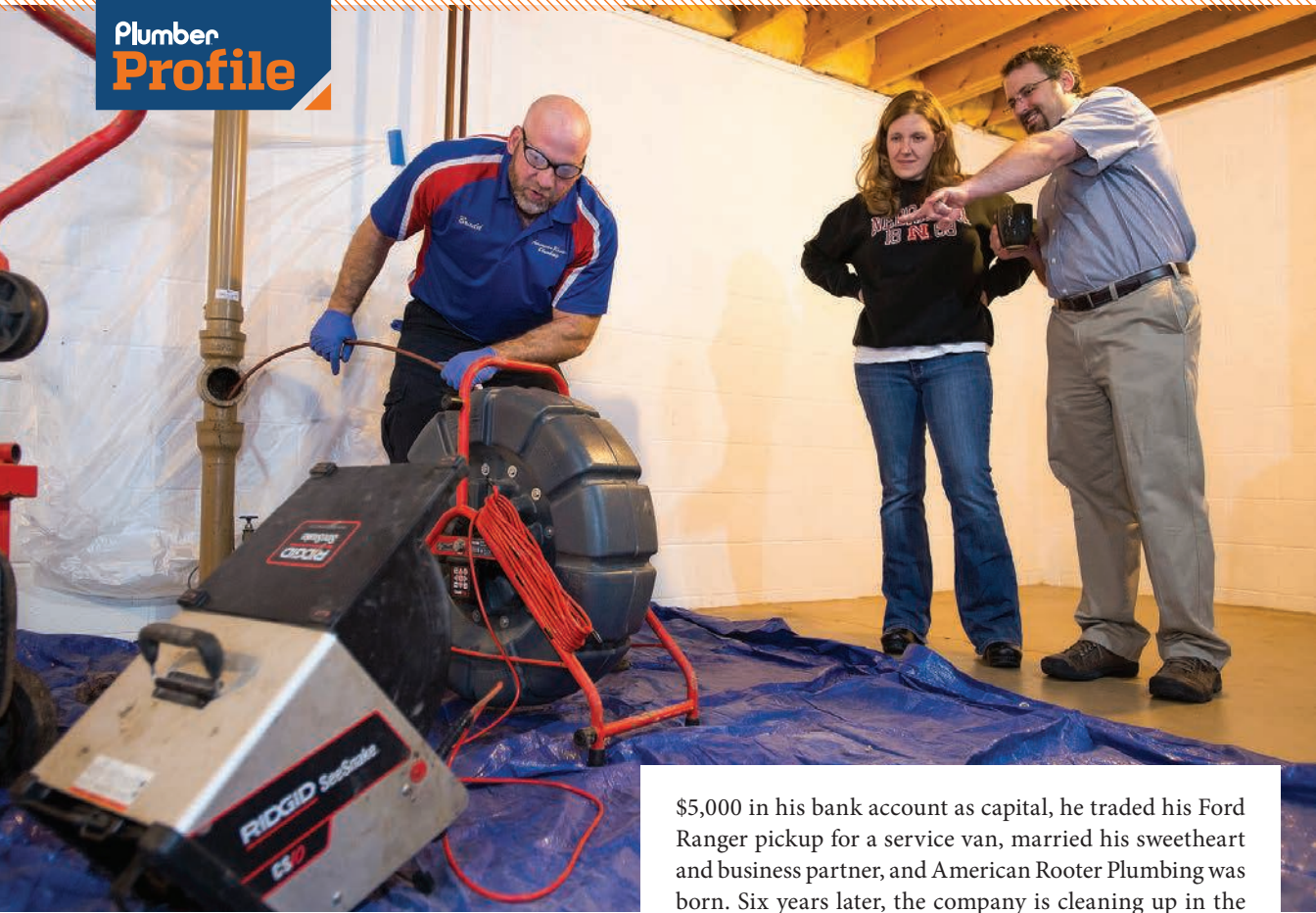
▲ Bradd Conn, master plumber and owner of American Rooter Plumbing, uses a RIDGID SeeSnake to observe the condition of the drain after a routine drain cleaning at a home in Omaha, Nebraska.
