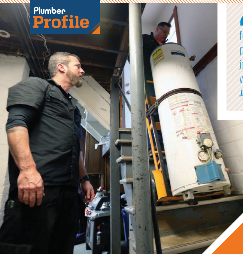
▲ Joel George, left, and Robert Werner, right, work together to change a hot-water heater at a residence. After draining and removing the previous tank, they installed a 40-gallon natural gas water heater.
