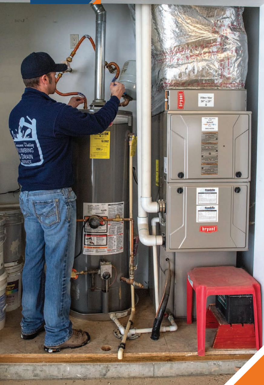
▲ Jeremiah Brown, Treasure Valley Plumbing and Drain Service technician, installs a Rheem water heater at a customer's home near Fruitland, Idaho.
