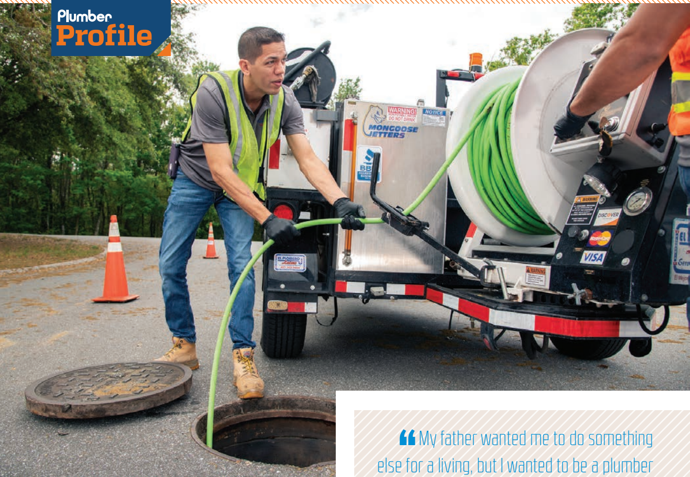
▲ Efesdamin Figueroa pulls out more hose from the company's Model 184 jetter (Mongoose Jetters by Sewer Equipment) to jet out a sewer line in Orlando, Florida.
