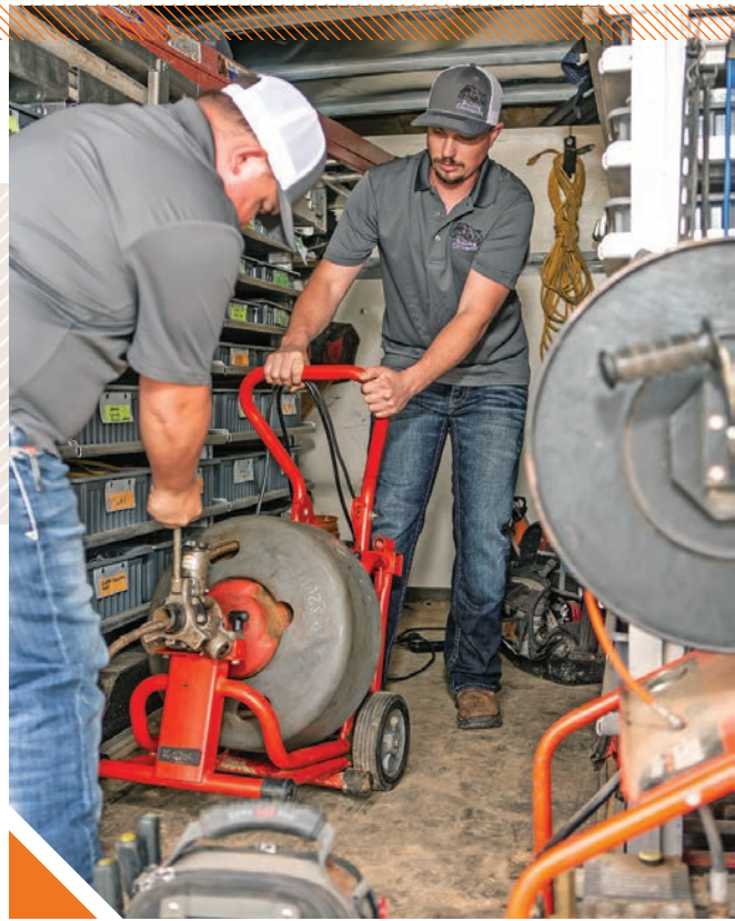
▲ Bulldog Contractors’ Jeff Keller, facing, and Cameron Corpier, plumber, unload a drum drain cleaning machine from a company van for a job site near Jefferson, Texas. The company vans are fully stocked with most supplies a plumber will need on a job.
