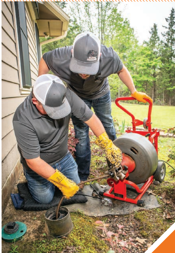
▲ While Cameron Corpier, kneeling, uses a RIDGID K-6200 drum machine to clear a customer’s mainline, Bulldog Contractors manager Jeff Keller checks in on the progress of the job.
