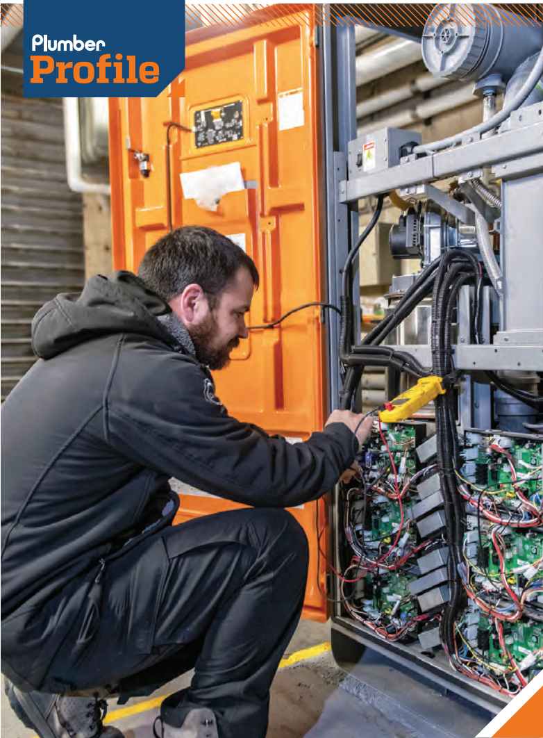
▲ Technician Brandon Content monitors a newly installed domestic tankless hot-water system by Intellihot.
