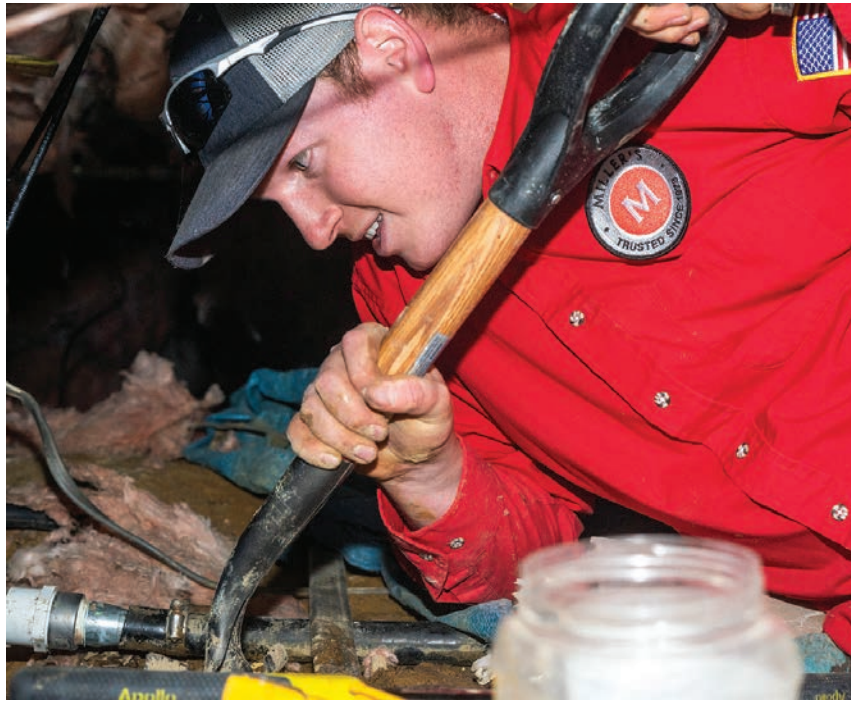
▲ Mark Nichols digs in a crawl space as he attempts to connect a water line to a pressure tank during the installation process.
