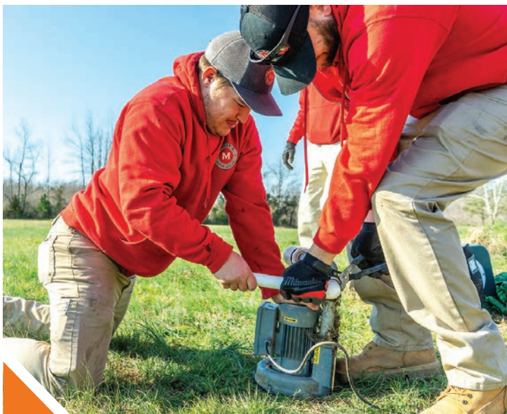
▲ Miller’s Services’ technicians Kenney Boyette, right, and Pierce Rained, left, replace pipe on the air pump from a septic system in hopes of repairing it. The company not only does plumbing service work, but also handles septic tank installation and pumping.
