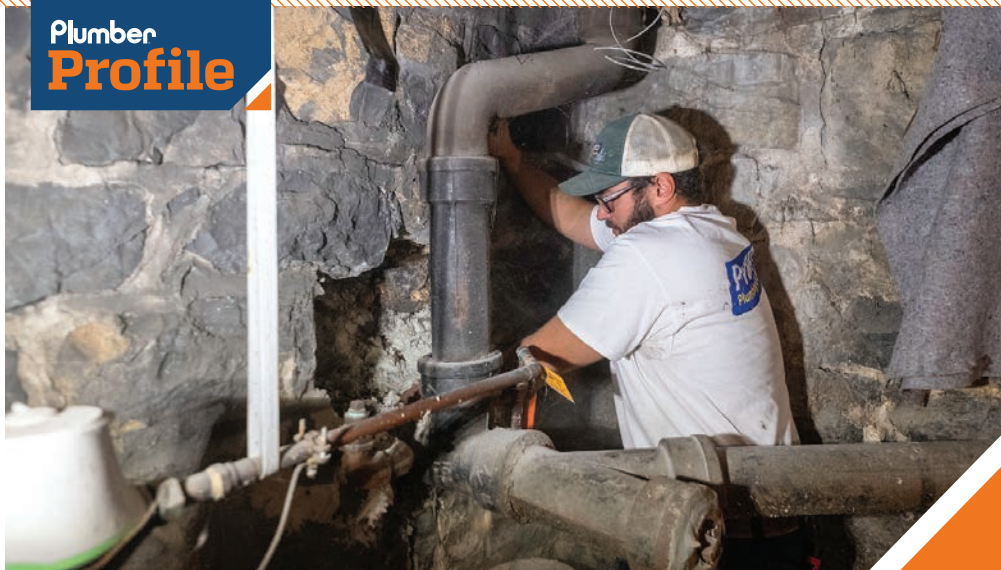
◀ Conner Trinkle begins the process of removing old sewer line that is being replaced in a home built in the late 1800s.
