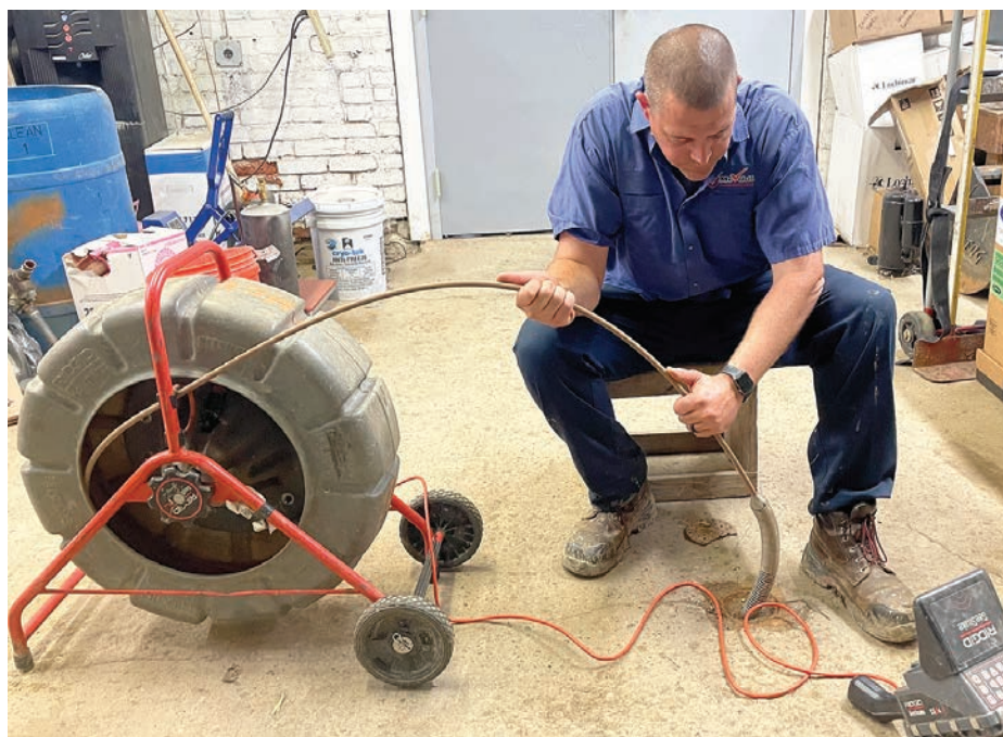
▶ Anthony Pacilla, vice president at McVehil Plumbing, Heating, and Air Conditioning, uses one of the company’s RIDGID SeeSnake inspection camera systems at a commercial property near Washington, Pennsylvania. (Photo courtesy McVehil Plumbing, Heating, and Air Conditioning)
