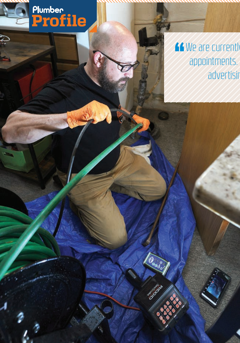
▲ The company often uses a Jetter Northwest Eagle 300 sewer jetting machine, to clean the sewer lateral of homes. Here, Chris Bontempo also uses a RIDGID SeeSnake to look at the inside of the pipe as he cleaned it out.
